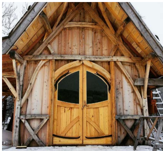
Vue de la façade Sud / view of the southern façade
