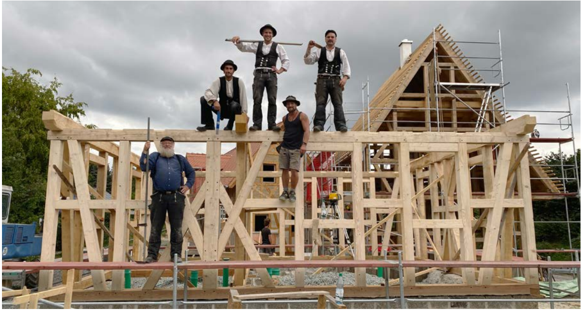
Les charpentiers montent le colombage / the carpenters assemble the half-timbering
